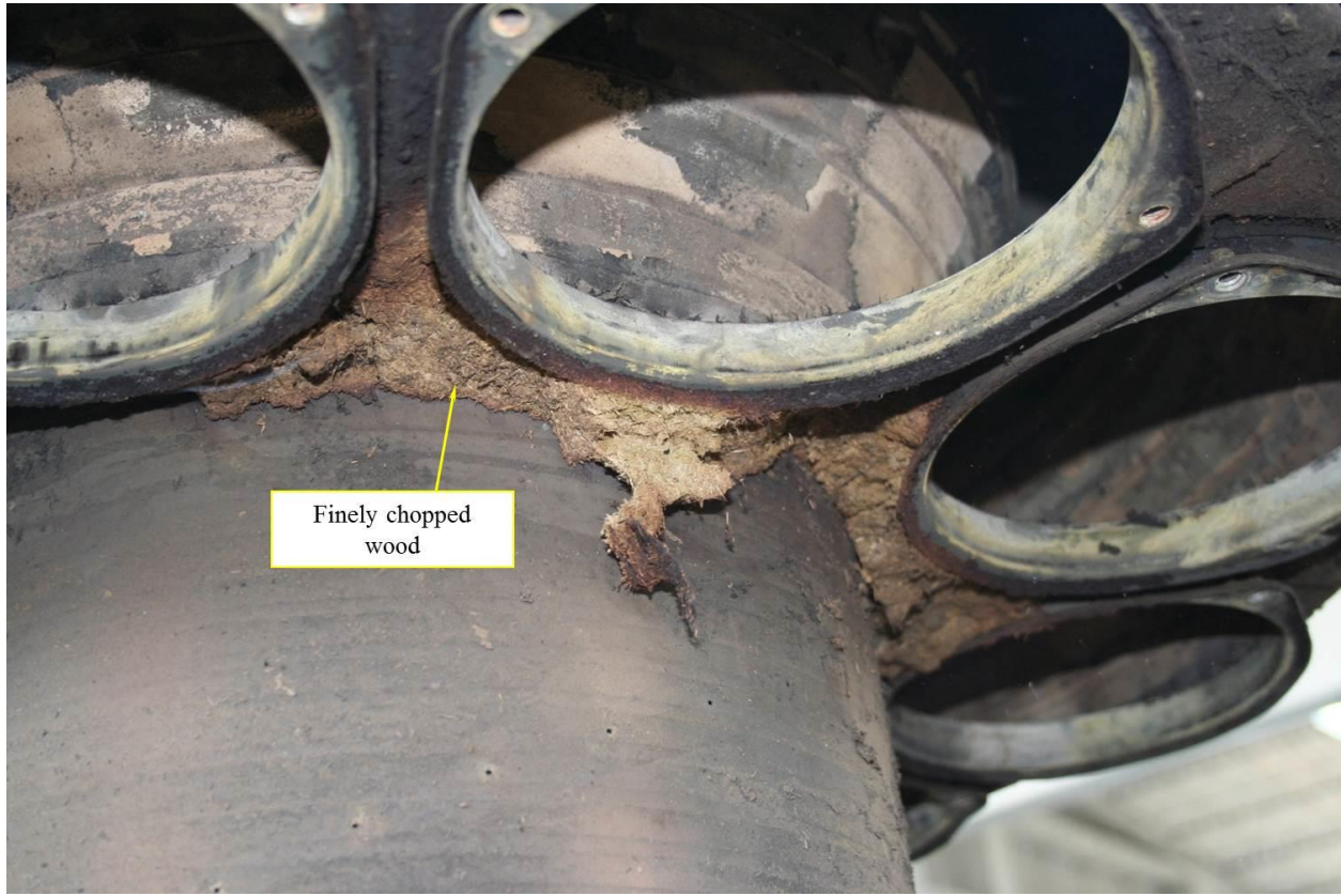
Figure 15: Deposited debris, including finely chopped wood fragments, deposited on combustion chamber support assembly
