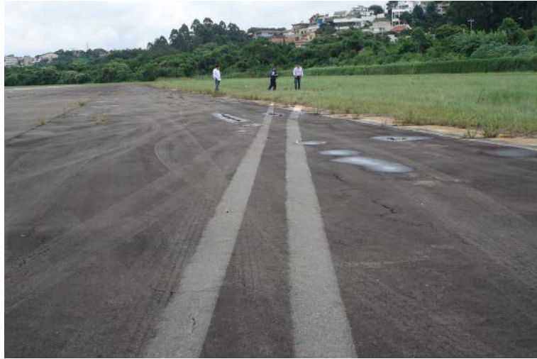
Figure 17 – Vapor marks left on the runway by hydroplaning tires (ref. 6)
