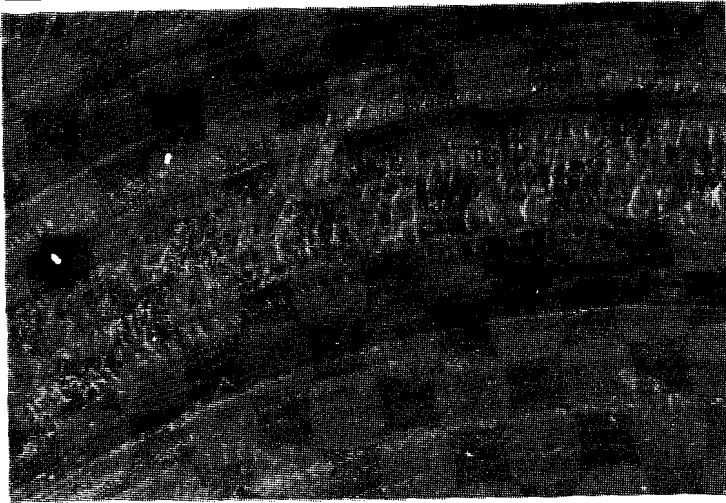
Figure 6 Enlarged Area of Figure 5 showing Fatigue Cracks
